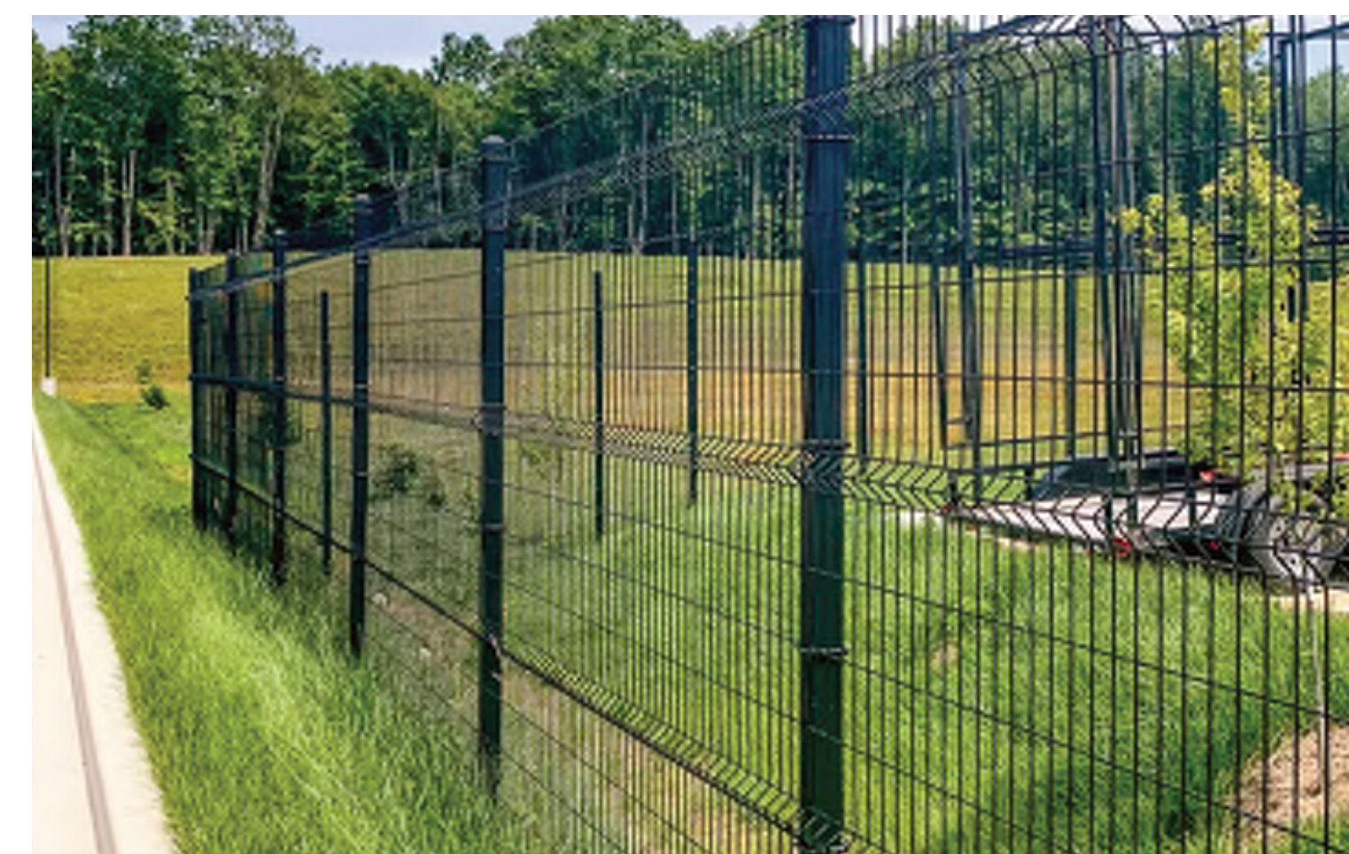
PANEL FENCE - REPAIR EXISTING AND EXTEND SW ADDITIONAL 350' TO SW (4' HT.)
